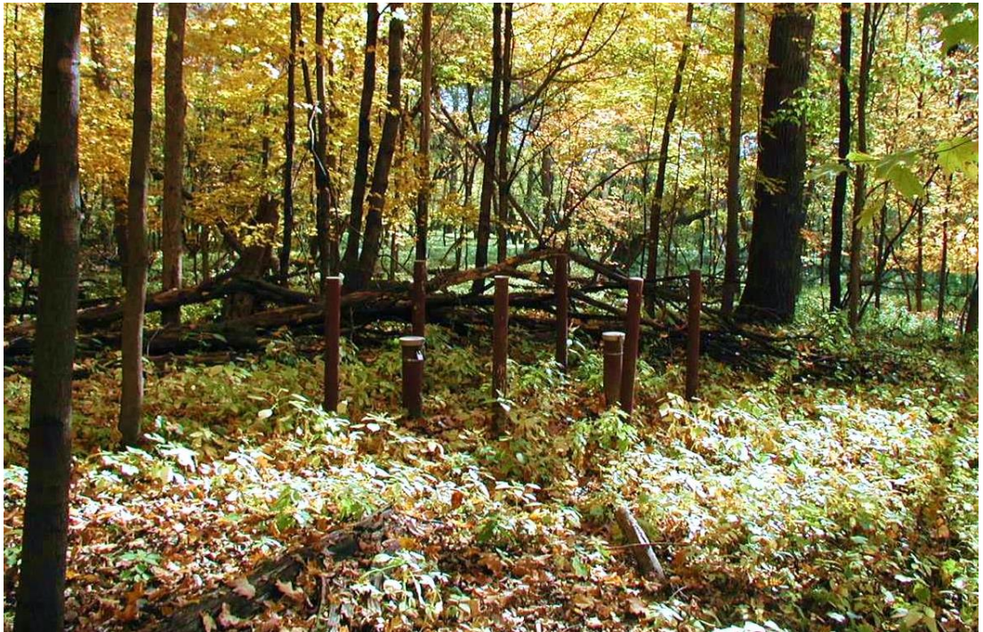
Photo: A nested well located in Seminary Fen used to monitor this groundwater dependent natural resource. This well is operated through a partnership between Carver County, the DNR, and the Lower Minnesota River Watershed District.
