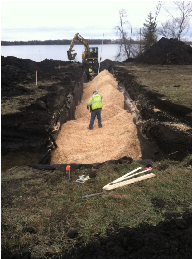
Bioreactor being installed—Hydes Lake in the background
