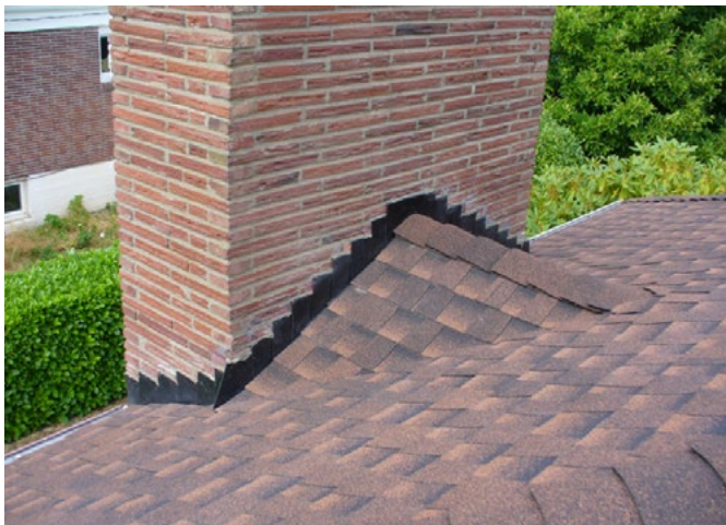
Cricket or saddle at chimney.
