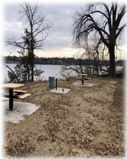
(Coney Island construction of picnic areas)
