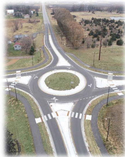
(Construction of CSAH 33 and 34 roundabout)
