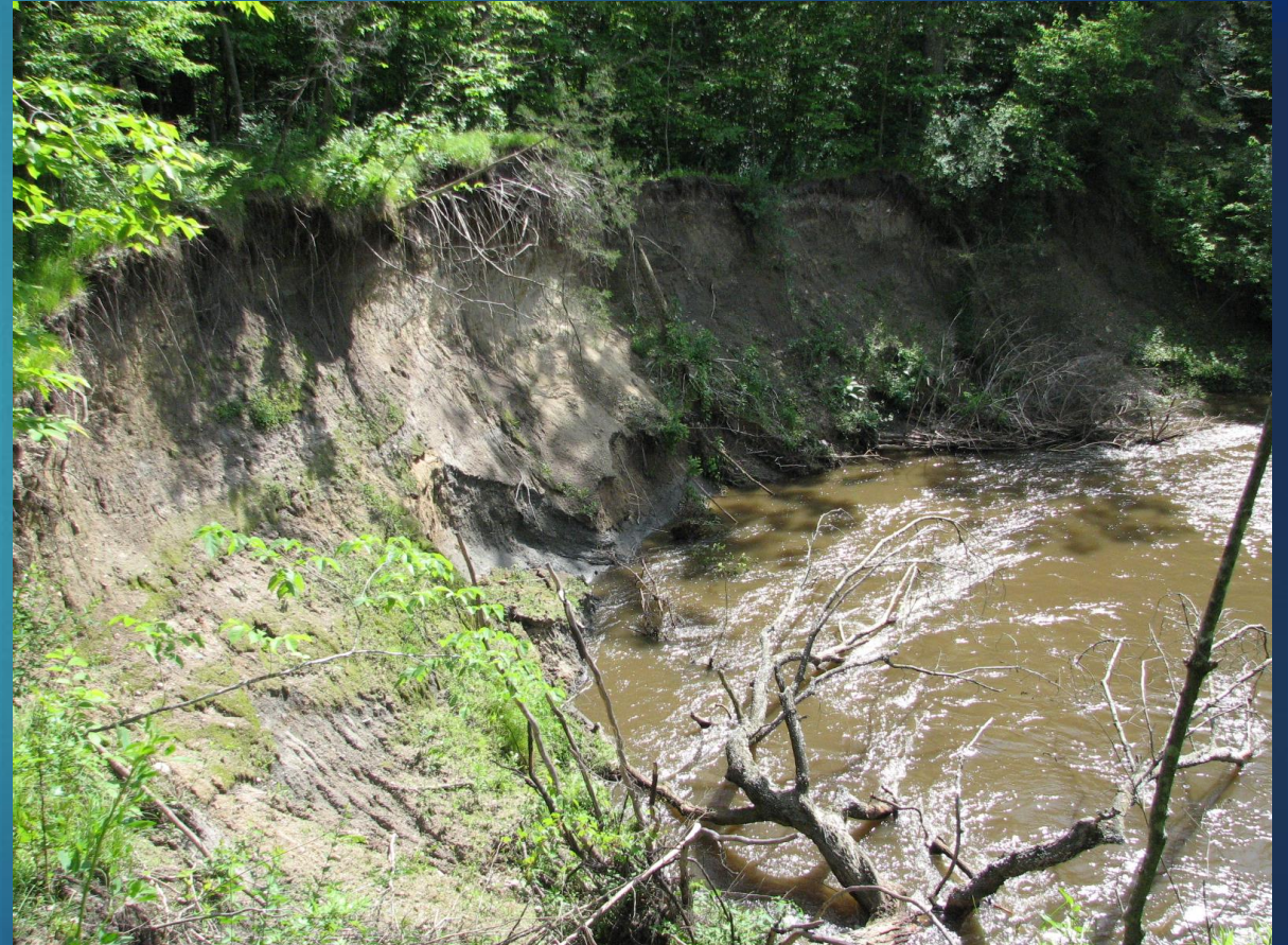
Bank erosion on Bevens Creek
