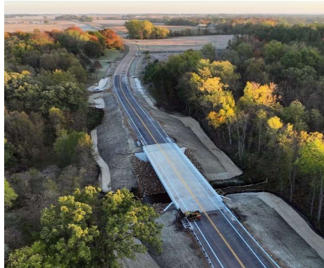
(CSAH 41 Bridge Project)
