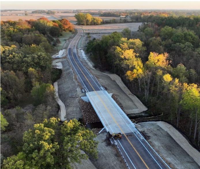
(CSAH 41 Bridge Project)
