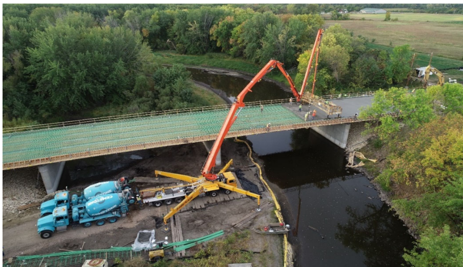
(Bridge replacement on CSAH 32 over South Fork Crow River)
