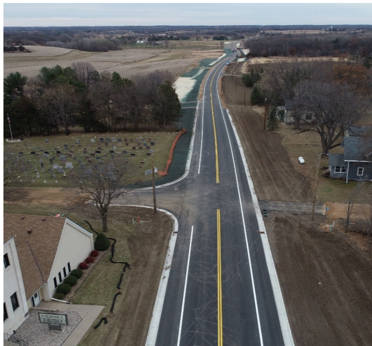
(Highway 24 Road improvements in the city of Watertown)
