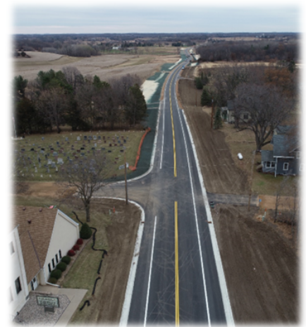
(Highway 24 Road improvements in the city of Watertown)
