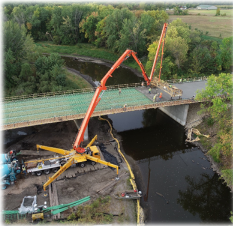
(Bridge replacement on CSAH 32 over South Fork Crow River)
