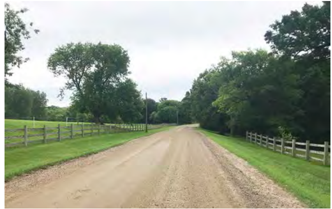
PHOTO: EXISTING CONDITIONS MARSH LAKE ROAD (RURAL)
