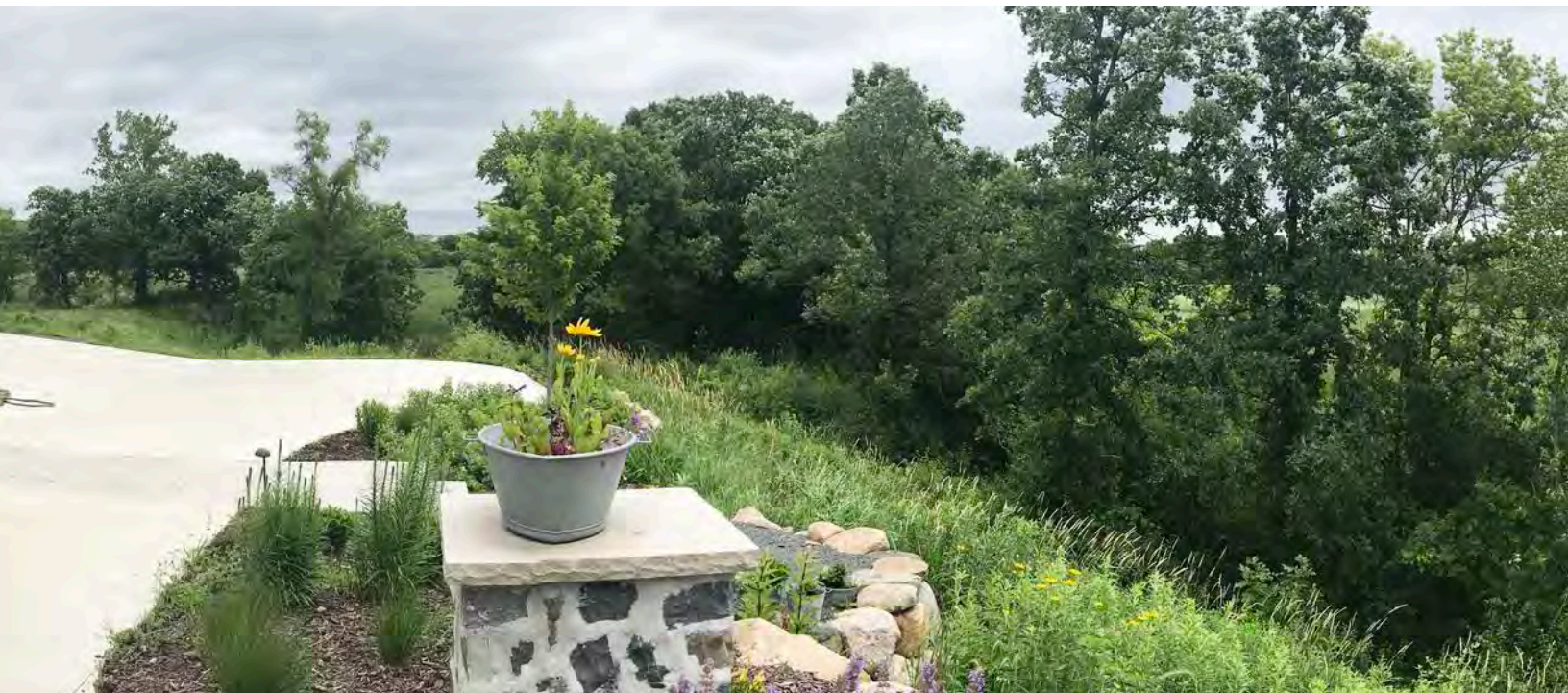
PHOTO: EXISTING CONDITIONS (HOUSING, STEEP GRADES & WETLANDS) OF PREVIOUS SWRT ROUTE FOR CONNECTION TO LMRT
