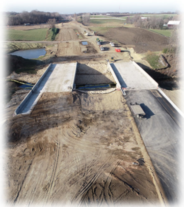
(Highway 212 construction in Dahlgren Township)
