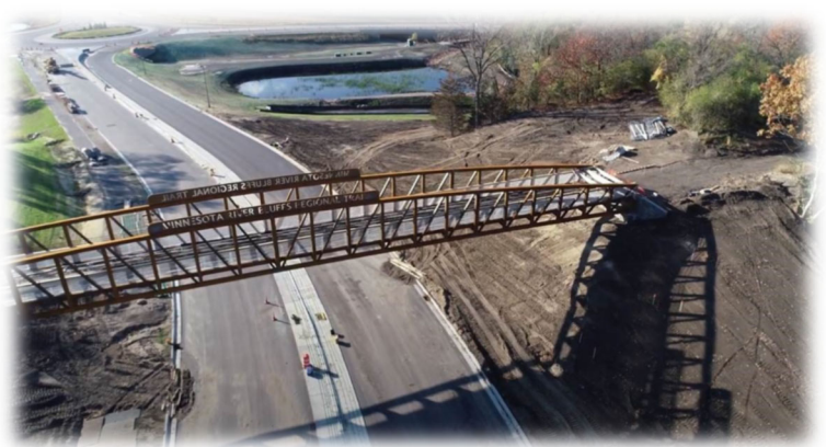
(Construction of Highway 101 and River Bluffs Regional Trail)
