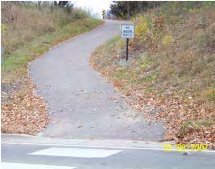
Looking west up at the western trail approach. The design of this approach forces trail users to navigate a 22 percent change in grade and then come to a complete stop at the roadway.
