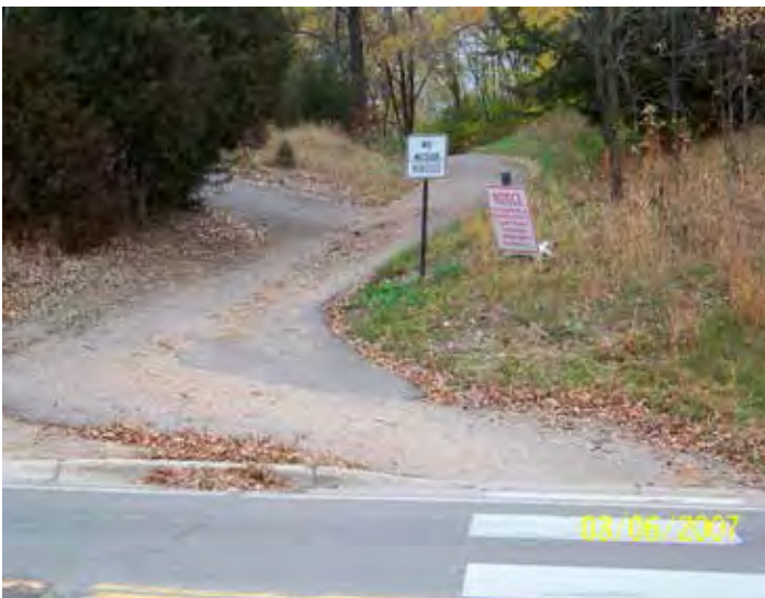
Looking up at the eastern trail approach. While not as steep as the western trail approach, trail users still have to navigate a steep descent and then come to a complete stop at the roadway.
