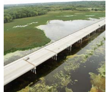
Highway 101 River Bridge. (Former TH 101)
